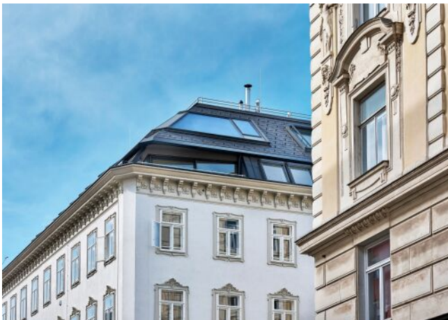
Essenz No. 1 | Fassade
