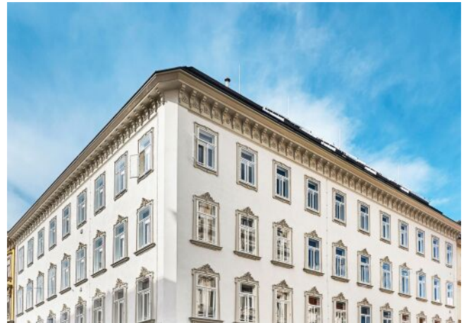
Essenz No. 1 | Fassade
