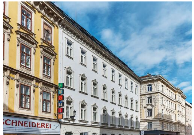
Essenz No. 1 | Fassade
