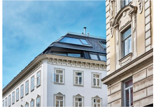
Essenz No. 1 | Fassade
