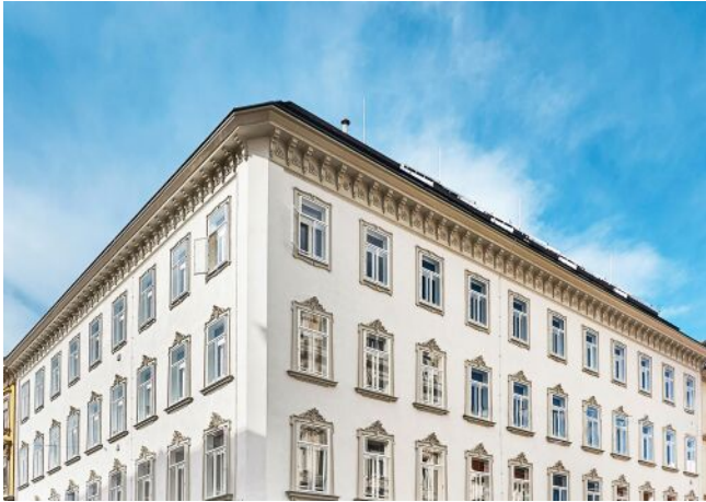
Essenz No. 1 | Fassade
