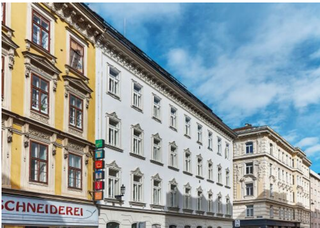
Essenz No. 1 | Fassade
