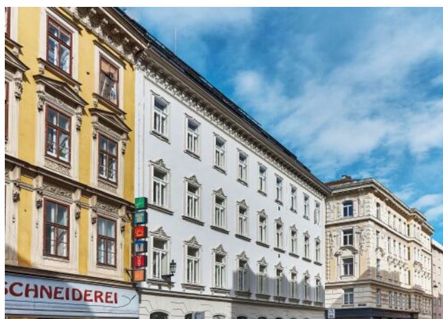
Essenz No. 1 | Fassade
