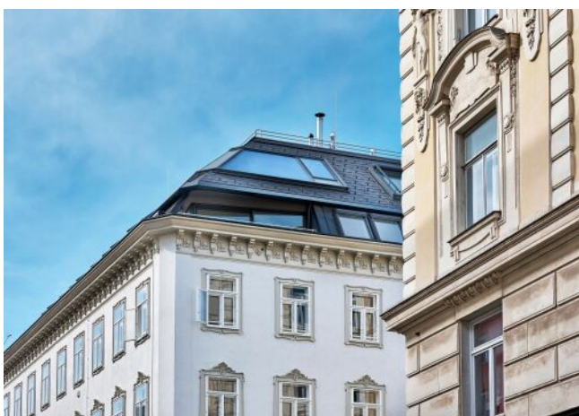
Essenz No. 1 | Fassade
