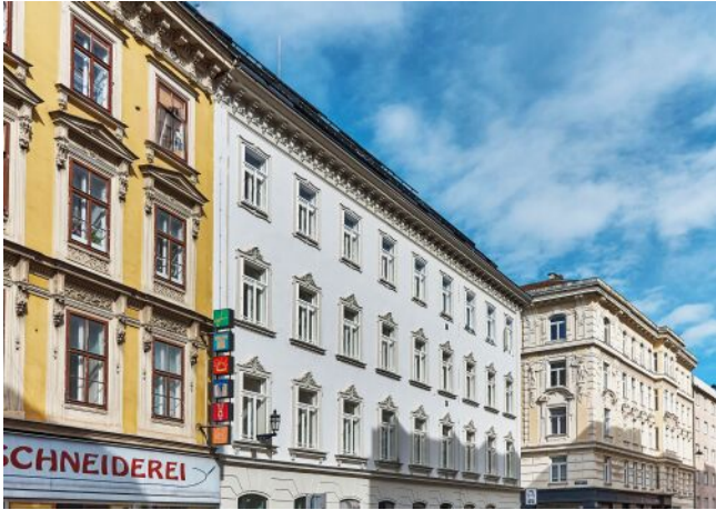
Essenz No. 1 | Fassade
