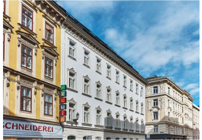
Essenz No. 1 | Fassade
