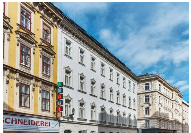
Essenz No. 1 | Fassade
