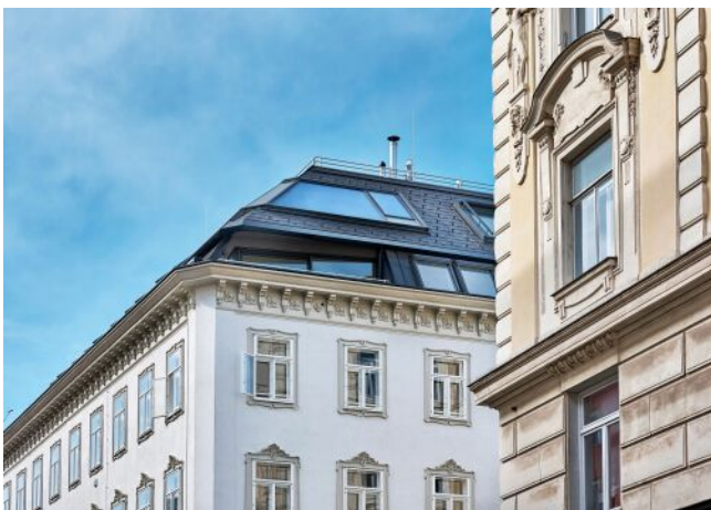
Essenz No. 1 | Fassade
