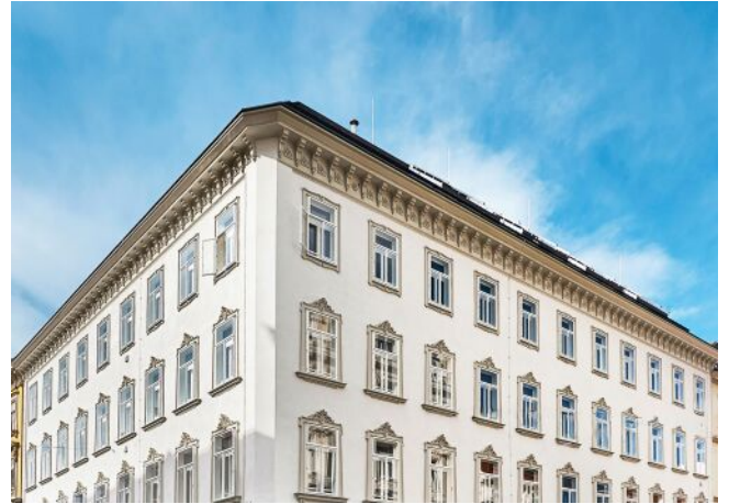
Essenz No. 1 | Fassade
