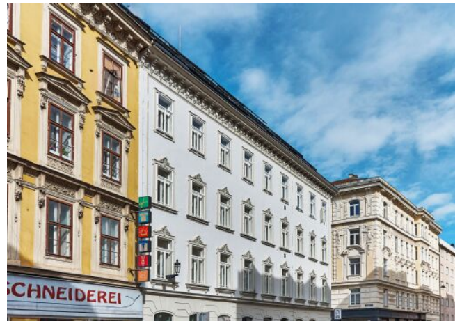
Essenz No. 1 | Fassade
