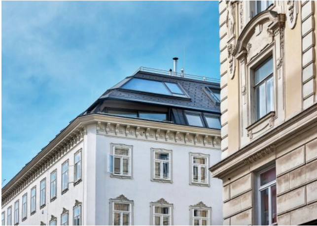
Essenz No. 1 | Fassade
