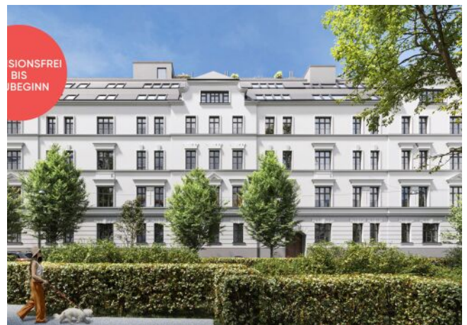
Roseggergasse | Fassade Frontal
