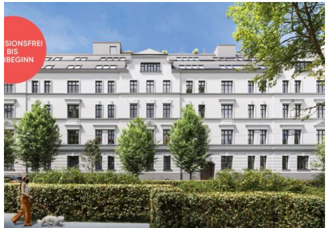
Roseggergasse | Fassade Frontal
