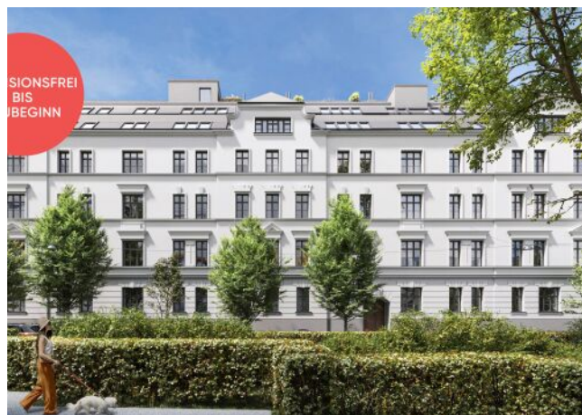
Roseggergasse | Fassade Frontal
