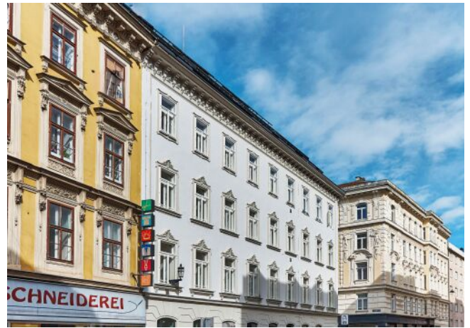
Essenz No. 1 | Fassade
