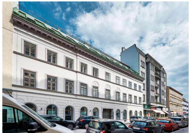
The Fusion | Fassade
