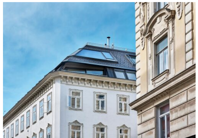
Essenz No. 1 | Fassade
