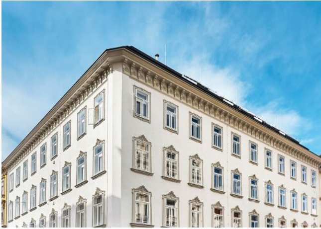
Essenz No. 1 | Fassade
